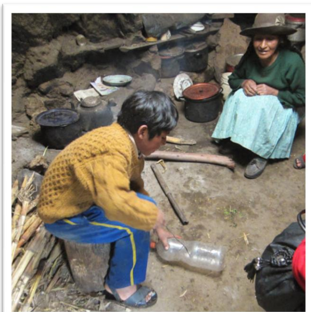
Yordi creating the new bottle strainer for the water pipe, using a wire heated in the lunch fire
