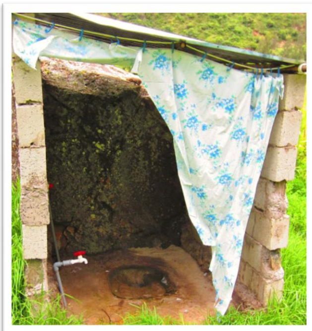
Has a shower head, standpipe and toilet platform
